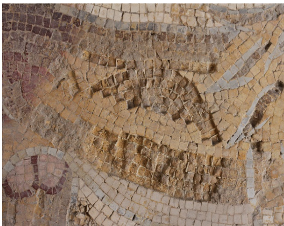
Figure 15. Tesserae deterioration( eroded tesserae)
