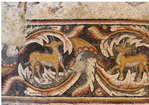
Figure 7. Lacuna filled with cement
