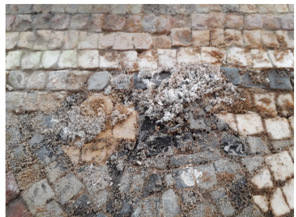
Figure 12. Efflorescence
