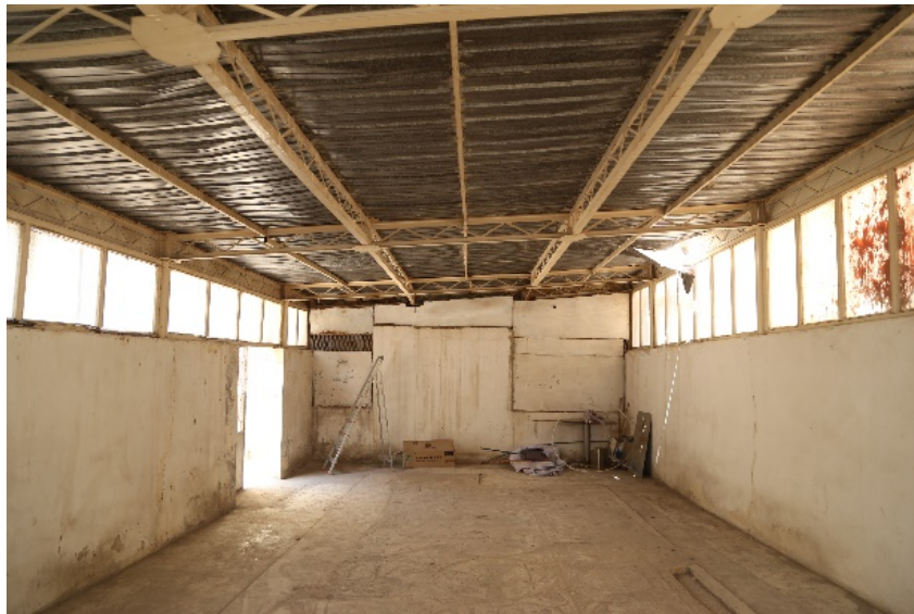
Figure 17. Holes and gaps in the roof
