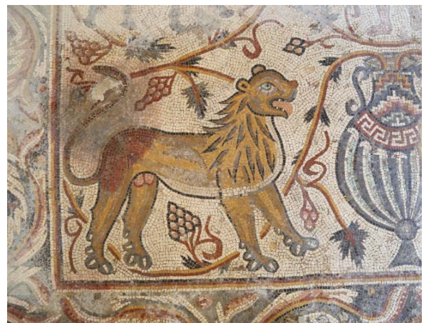
Figure 16. Color alteration (fire damage)
